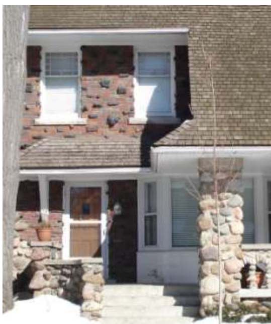
Figure 3.21 Rusticated brickwork with a rubble stone veranda – 25 Munro Park Ave. March 2008
