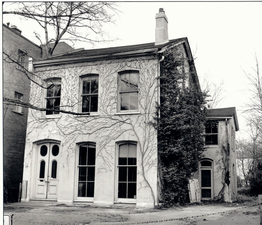
#10 Prince Arthur Avenue façade (1991)
