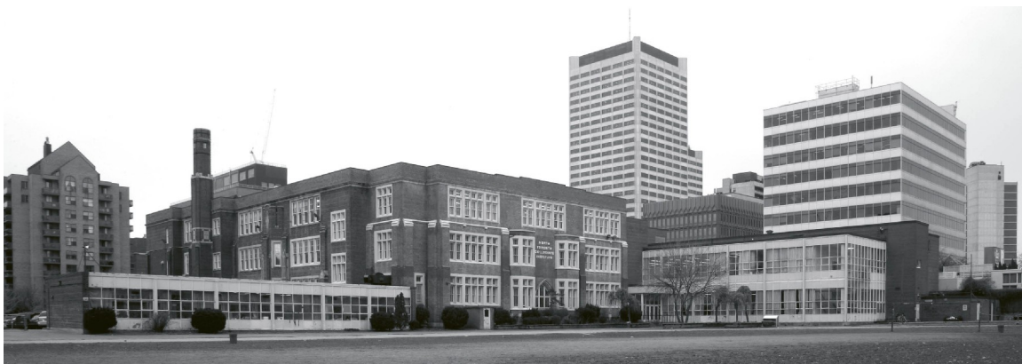
View from Broadway Avenue, showing the east (left) and north (right) elevations of the 1912 building at North Toronto Collegiate Institute (date: 2007)
