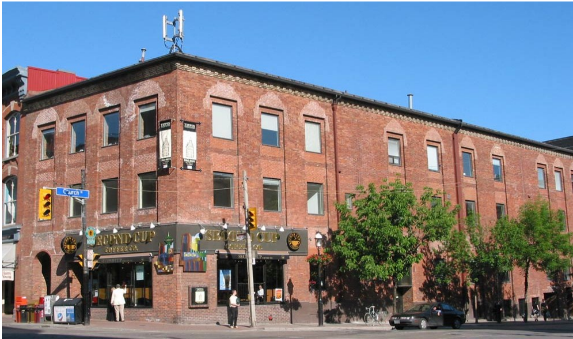
Corner View: North (Front St E) and West (Church St) Elevations
