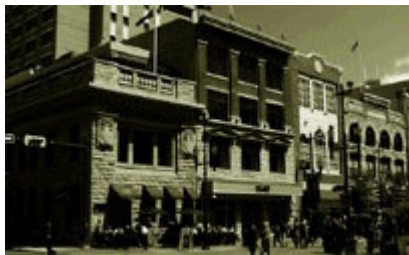
This addition to a bank in Calgary, Alberta was built as a greenhouse type rooftop structure set back from the wall plane. The existing high parapet, making it as inconspicuous as possible from the street, largely conceals it. While distinguishable from the elaborate sandstone exterior of the original building, it is physically and visually compatible, and subordinate to, the historic building.
