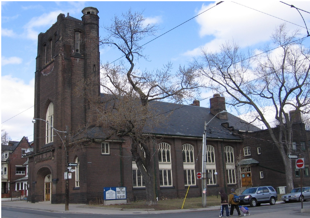
West façade on Broadview Avenue (left) & south elevation on Simpson Avenue (right)
