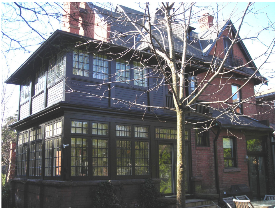
View looking at side and rear elevations of the sun porch
