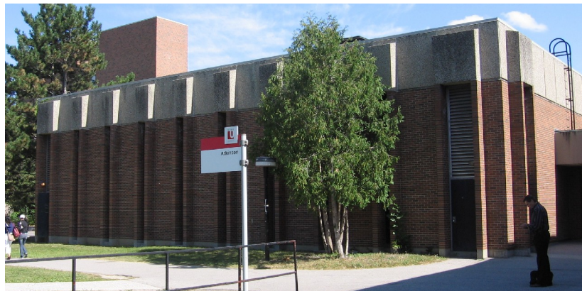
Phase I, Elvira Elliott Atkinson Hall (west façade shown)
