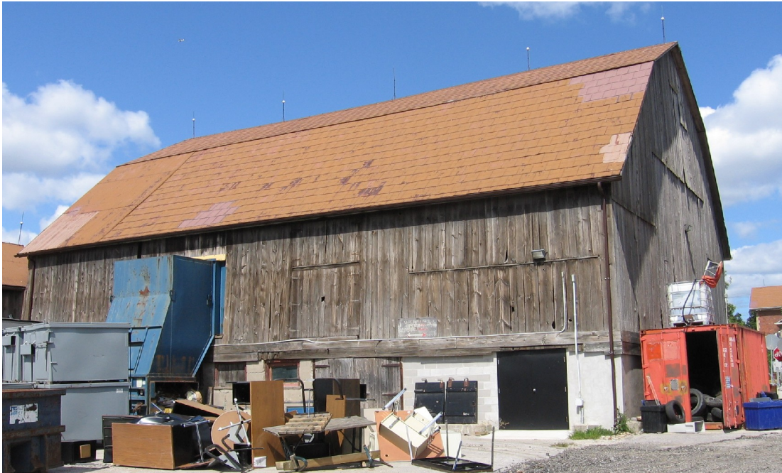
Jacob Stong Barn, showing south elevation
