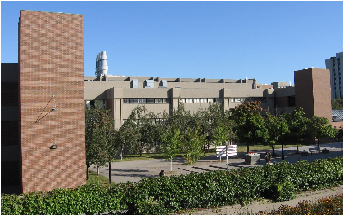
Farquharson Life Sciences Building, showing south elevation
