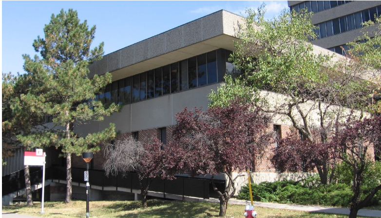
Phase I academic building (west & south facades shown)
