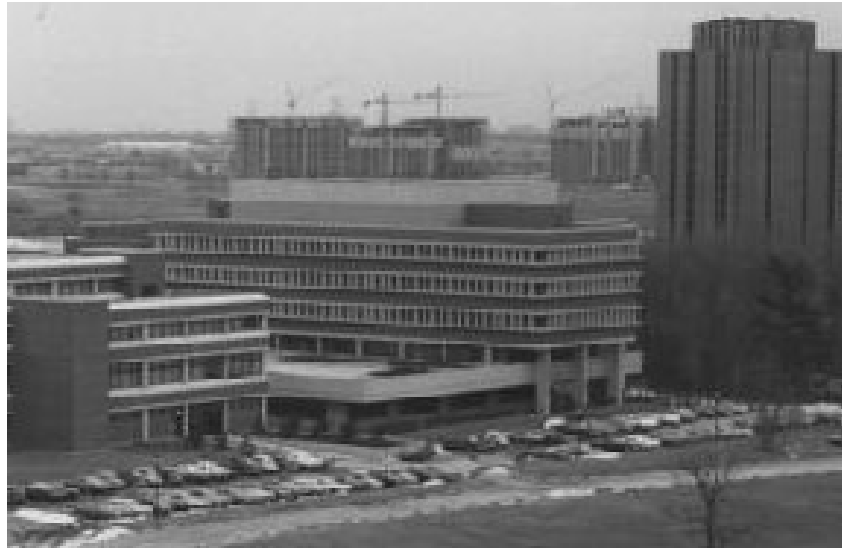
Osgoode Hall Law School (centre), undated, view from northwest (Source: Archives, York University, http://pi.library.yorku.ca/dspace/handle/10315/1127 )
