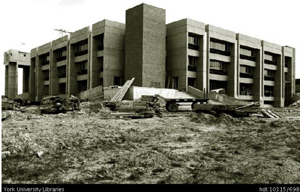
Petrie Science and Engineering Building, 1968, showing west elevation and observatory (left), with south elevation (right) (Source: Archives, York University, http://pi.library.yorku.ca/dspace/handle/10315/698 )
