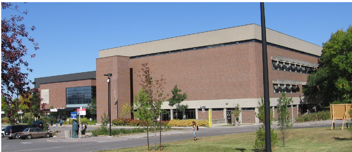
Tait McKenzie Centre, Phase I, showing south elevation (left)
