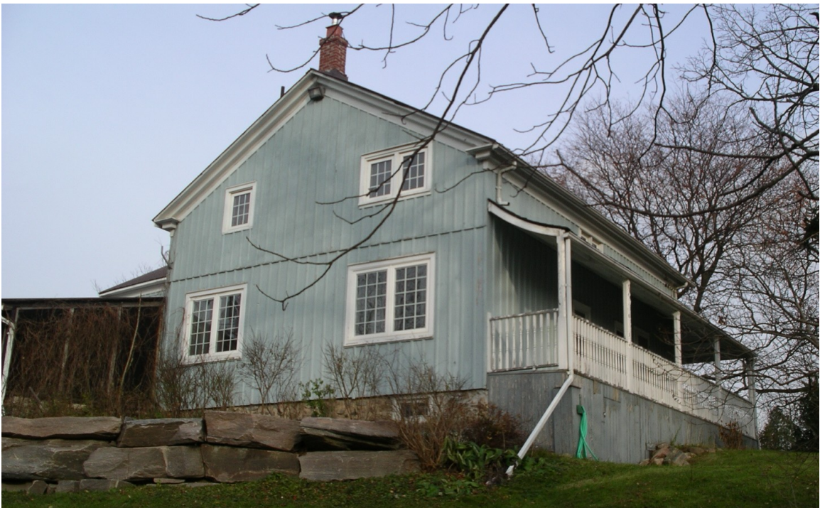
West façade (right) and north elevation (left)
