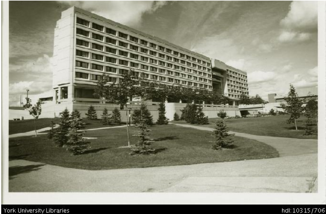
Ross Building, undated, showing south (left) and east (right) elevations (Source: Archives, York University, http://pi.library.yorku.ca/dspace/handle/10315/706 )
