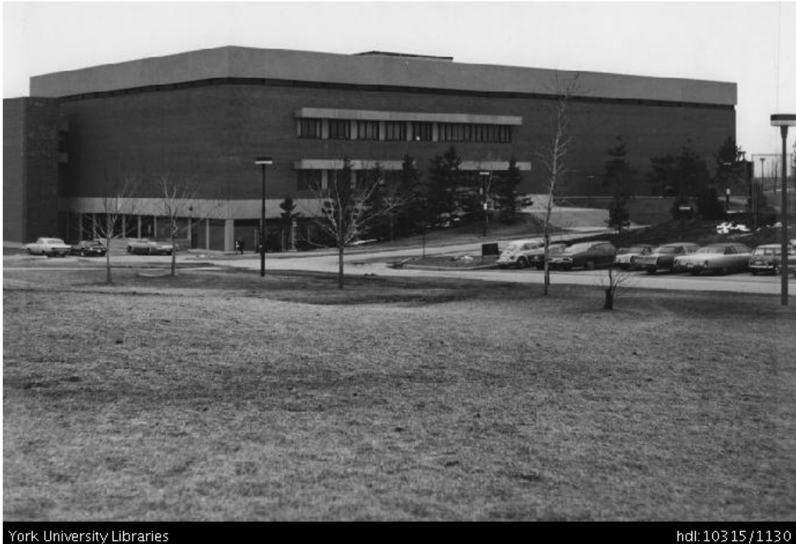
Tait McKenzie Centre, Phase 1, undated, showing south (left) and east (right) elevations (Source: Archives, York University, http://pi.library.yorku.ca/dspace/handle/10315/1130 )
