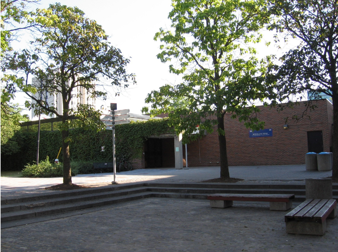
Stedman Lecture Halls, showing west elevation and entrance
