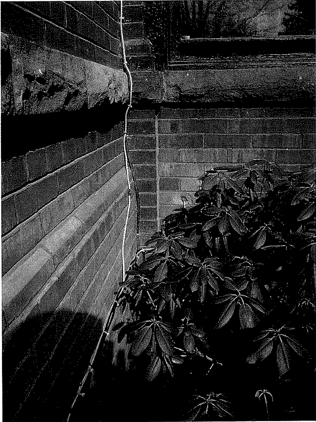
Figure 13 . Plinth Stone. Source: ERA Architects
