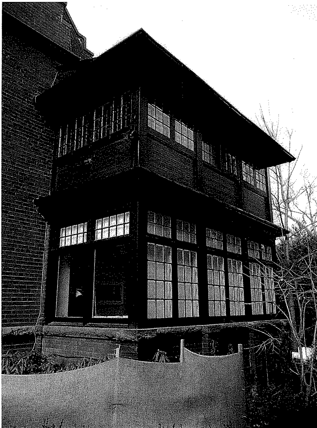
Figure 5. Sun Room. Source: ERA Architects
