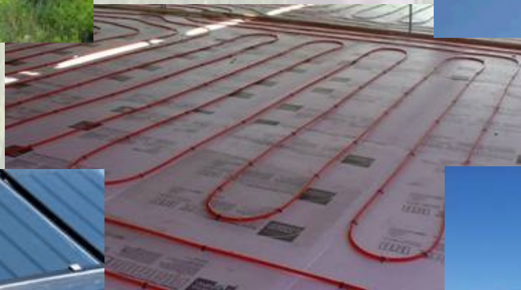
Radiant Floor Heating
