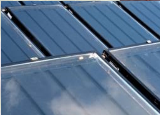
Solar Water Heater
