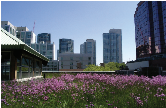
Example of planted green roof treatment.
