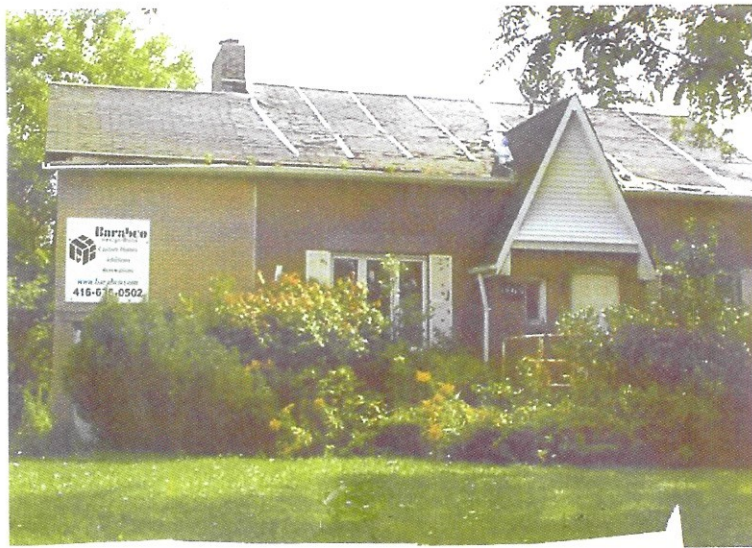
FRONT ELEVATION. SEE CONDITION OF ROOF.
