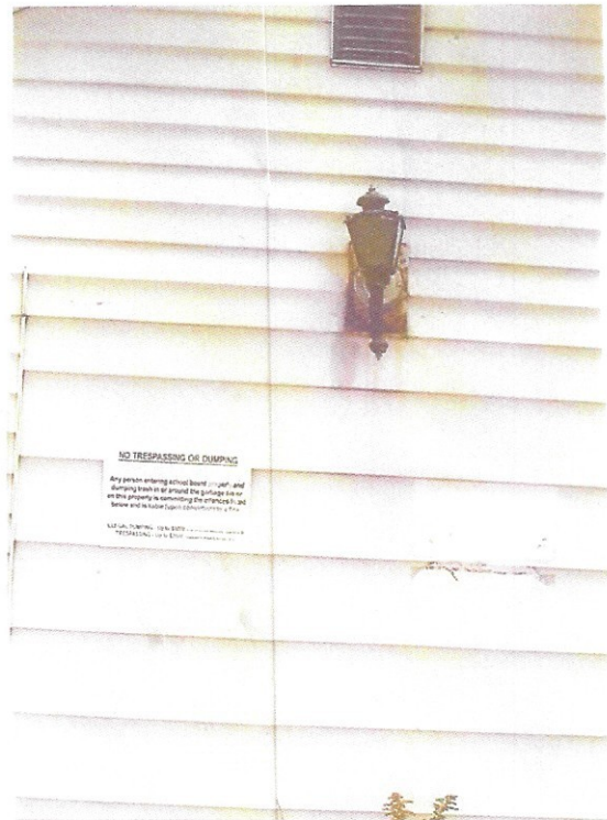
WARNING SIGN AT THE FRONT.
