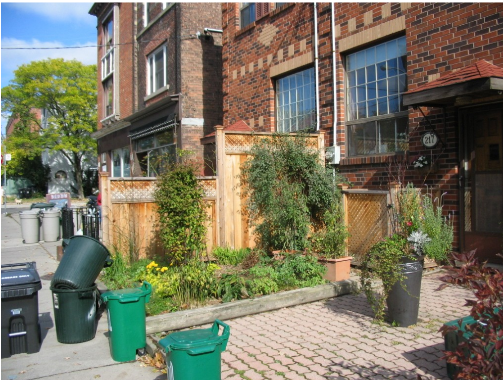
217 Sorauren Avenue facing north – October 22, 2008
