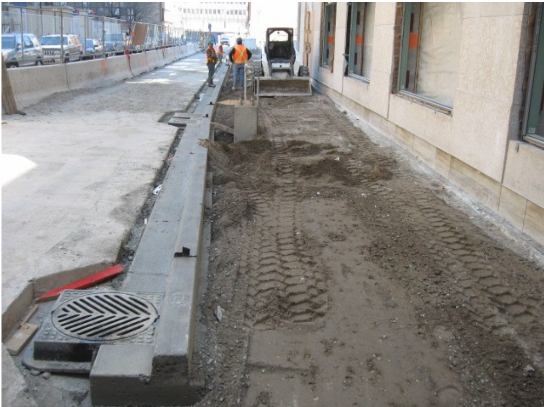
40 Adelaide Street West – Temperance Street flank April 16, 2009
