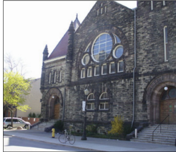
(right) Robert Street Face of Trinity-St. Paul United Church, adjacent to the District
