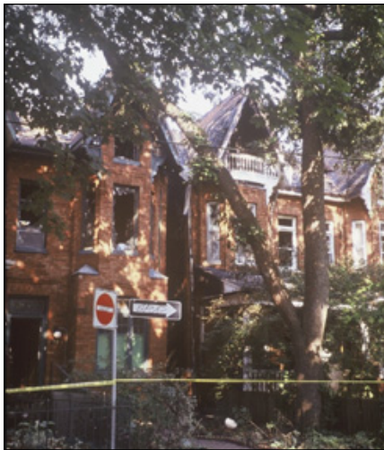
Nos. 52-60 Robert Street, built by Frederick Clements, seen here shortly after the recent fire.
