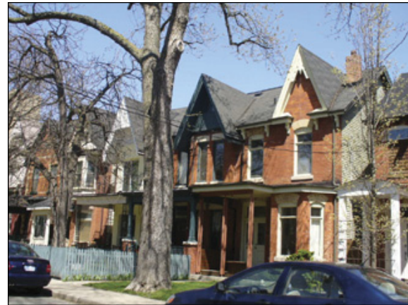
Row near 105 Robert Street (1886), with bracketed overhang and simple gables. The “bay” just on ground floor, porches have been replaced.
