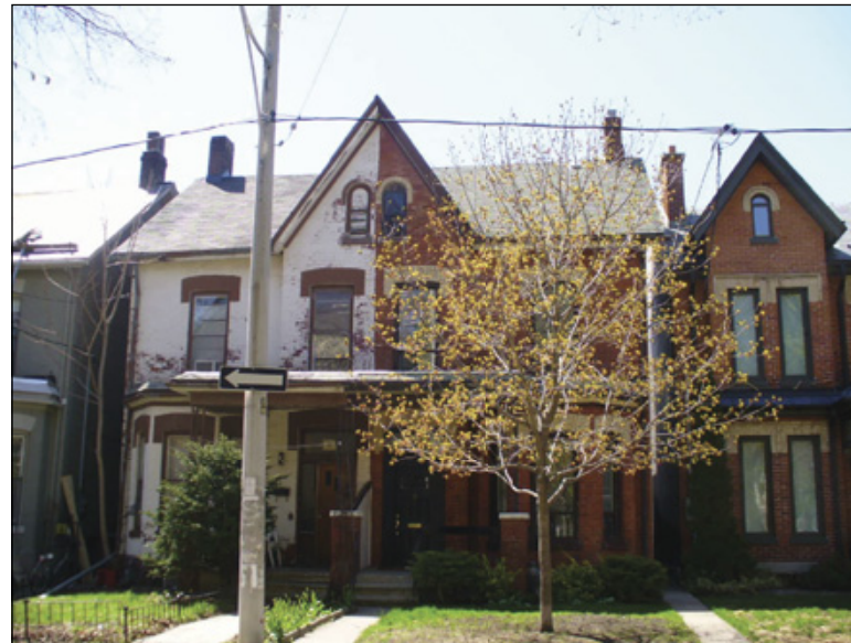
Houses by William McBean, 1884, close the view from Willcocks Street
