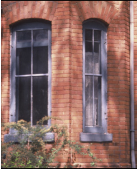
Restored wooden storm window (Cabbagetown example)
