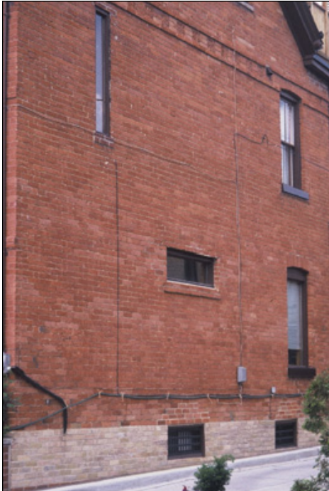
Restored Brickwork at No. 1 Laurier Avenue in Cabbagetown
