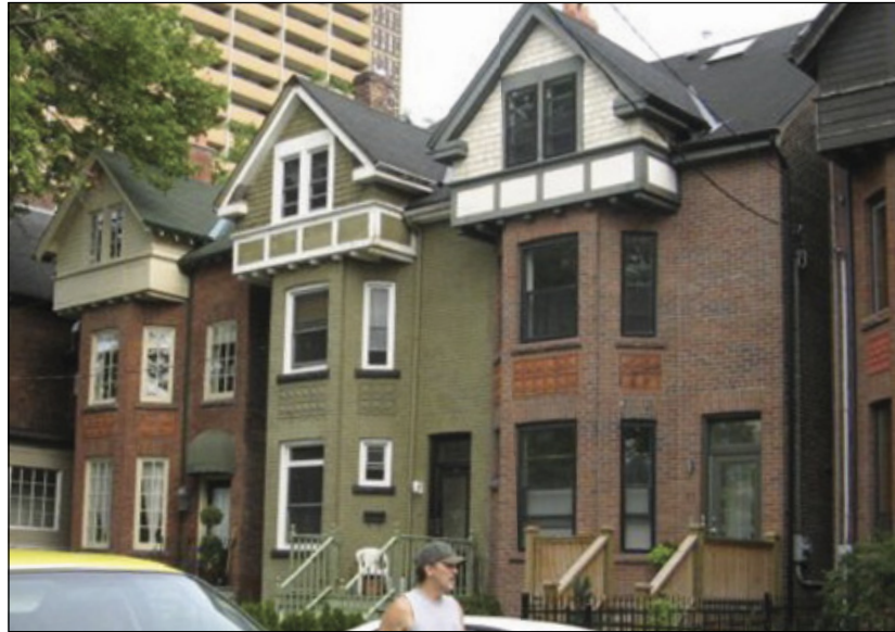
Houses on Sussex Avenue designed by C.R.S. Dinnick, 1900
