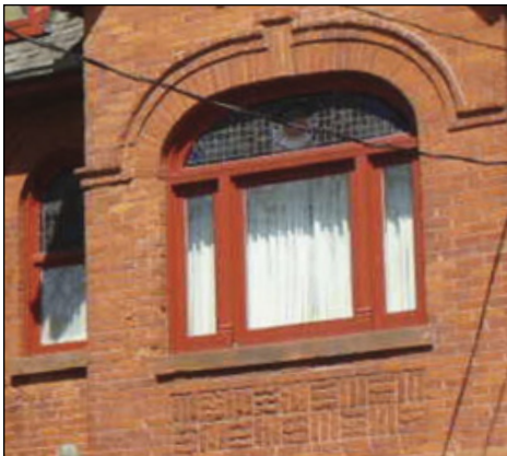
Stained glass windows are common features on “Bay-n-Gable” houses, also note the decorative brick inset panel
