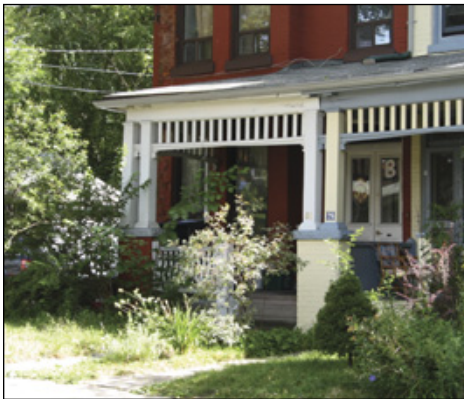
Small porch tucked between Bays is typical of the Victorian porches, after 1900 many houses added larger porches with brick piers, heavier porch posts.
