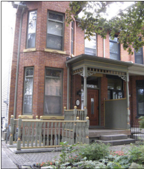
A good example of a basement entrance, designed in character with and also preserving the porch details. (built before these guidelines were issued)
