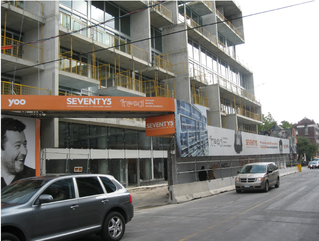
Fronting 75 Portland Street
