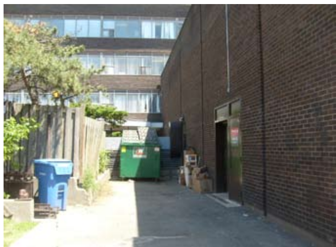
Loading and servicing should be more thoughtfully considered
