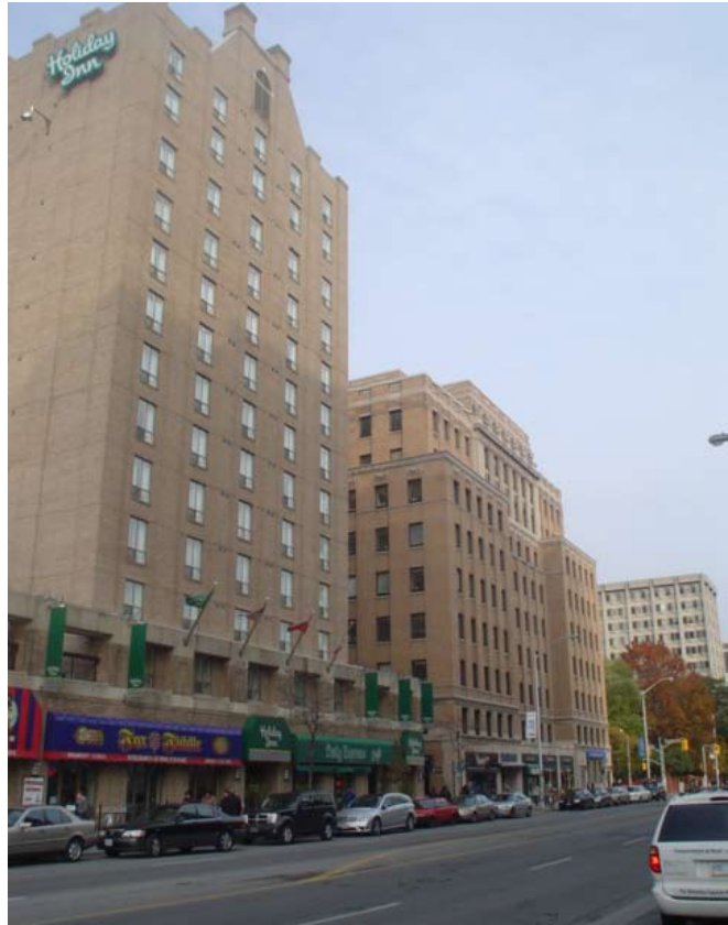
Articulation of building elements - Institutional Precinct
