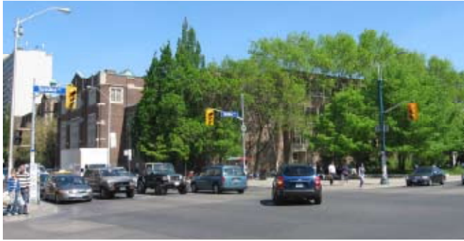
UTS building at Southeast Corner
