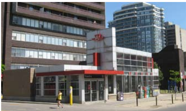
TTC entrance at Walmer Road
