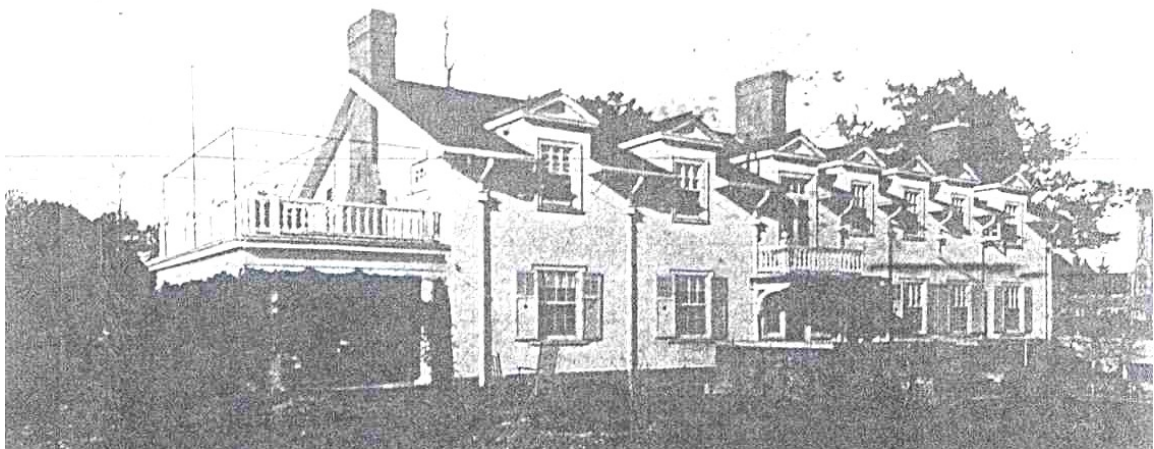
Photograph, John B. Maclean House (1910), showing the south elevation (source: Construction , November 1911, 52)
