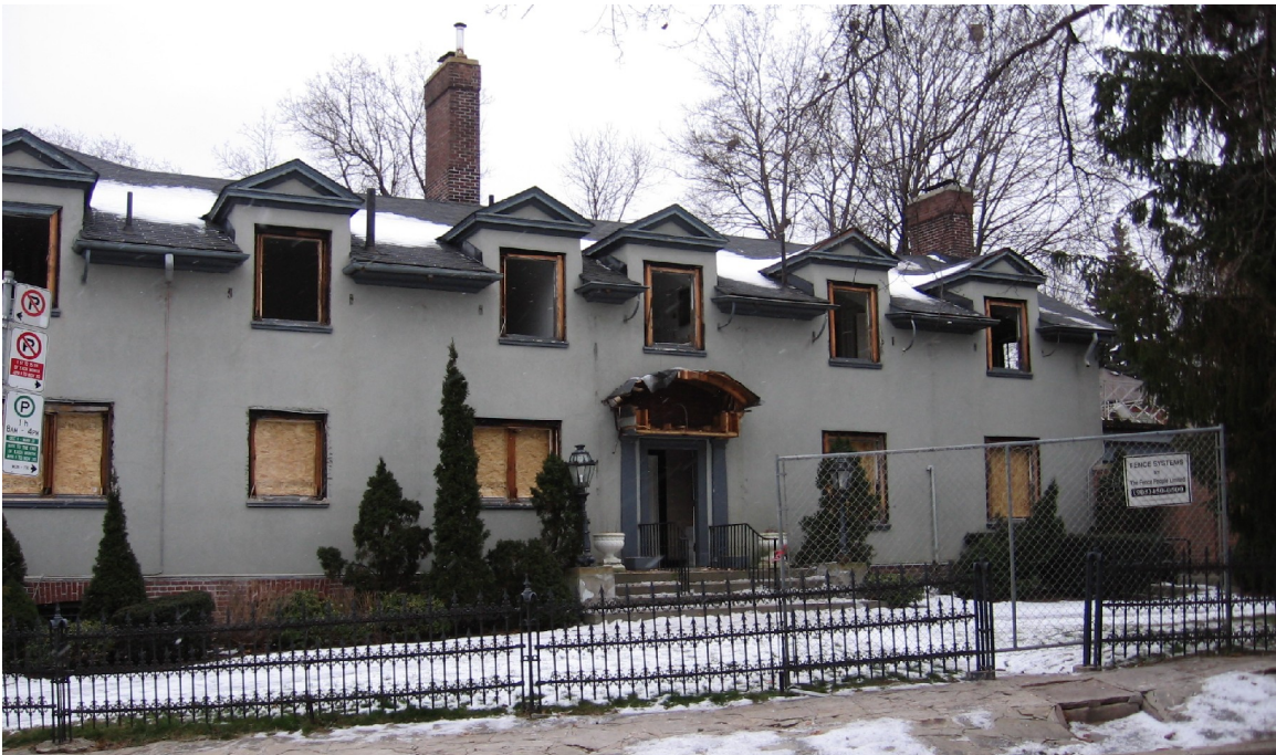
Principal (north) façade, December 2009, following alterations
