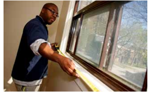
Cleaning and preparing a vacant unit for a new tenant in the Pelham Park townhomes.
