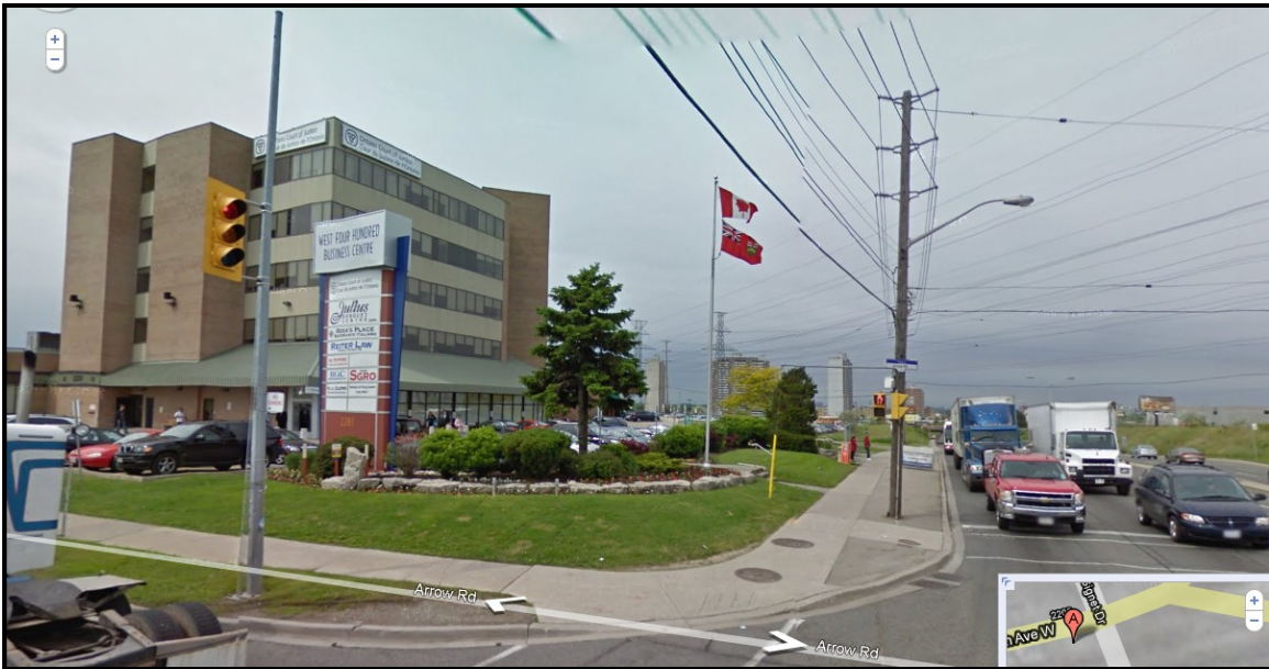
North end of the property at 2201 Finch Ave.W. Intersection of Arrow Rd. and Finch Ave.W.
