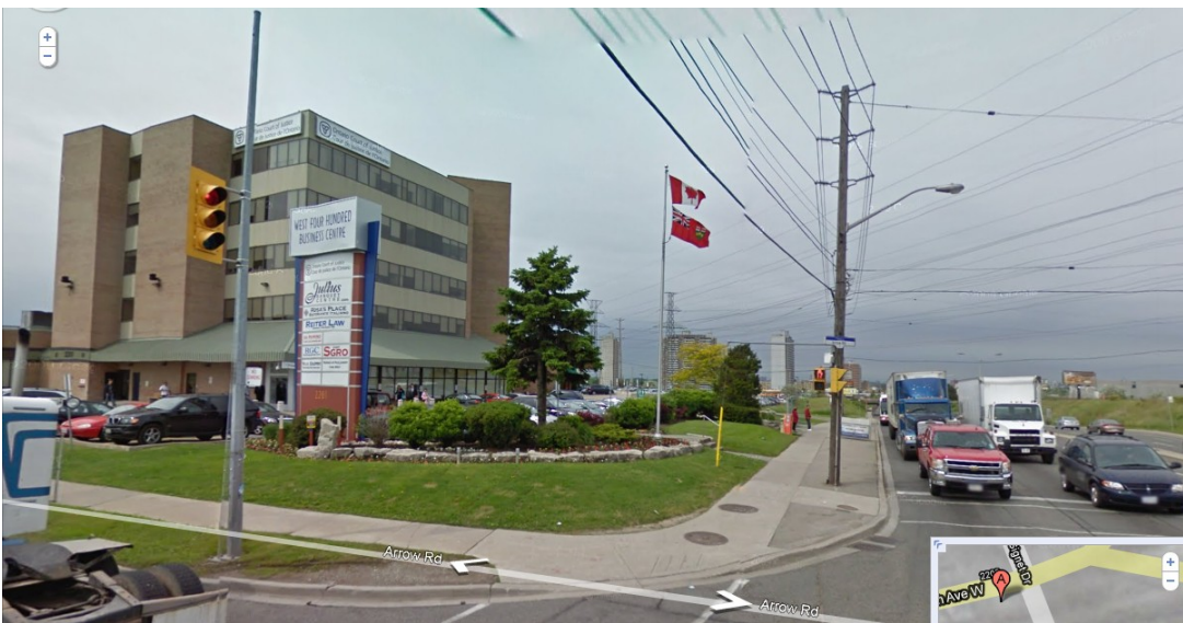
North end of 2201 Finch Ave W looking west along Finch Ave W
