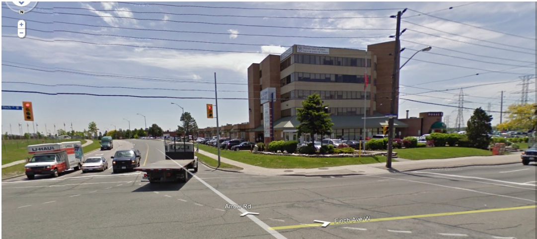
North end of 2201 Finch Ave W
