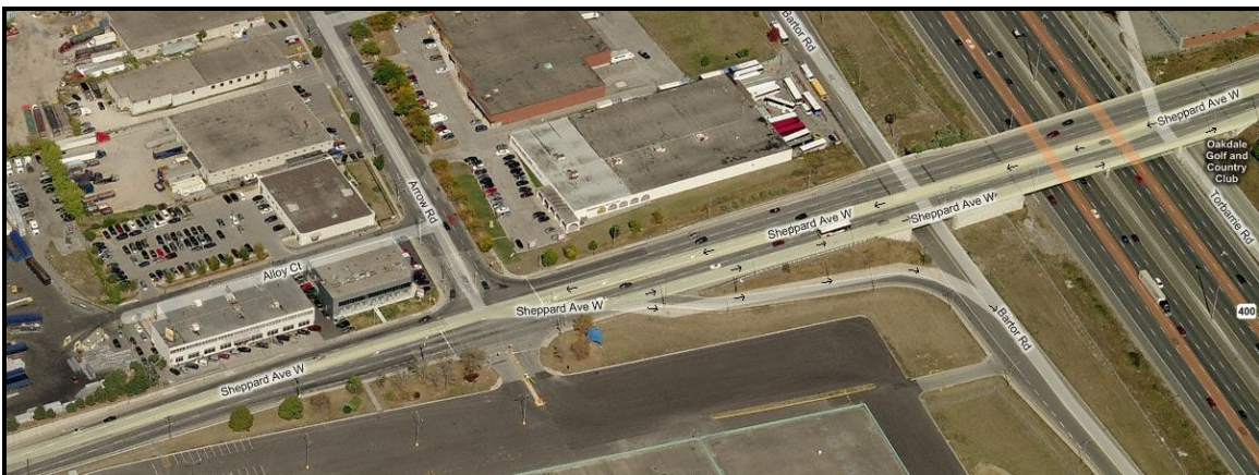
Aerial view of the area in around 2250 Sheppard Ave W
