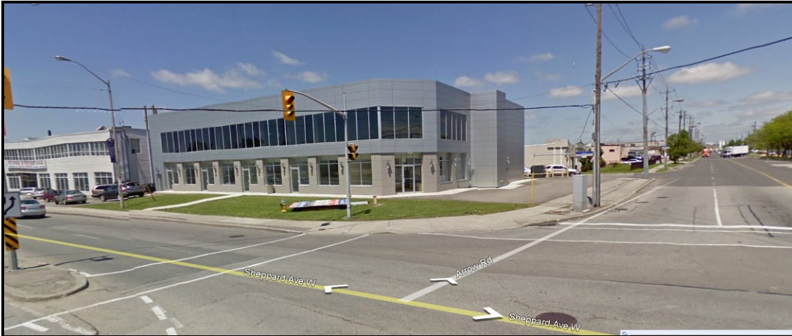
South - east elevations at 2250 Sheppard Ave W looking north.
