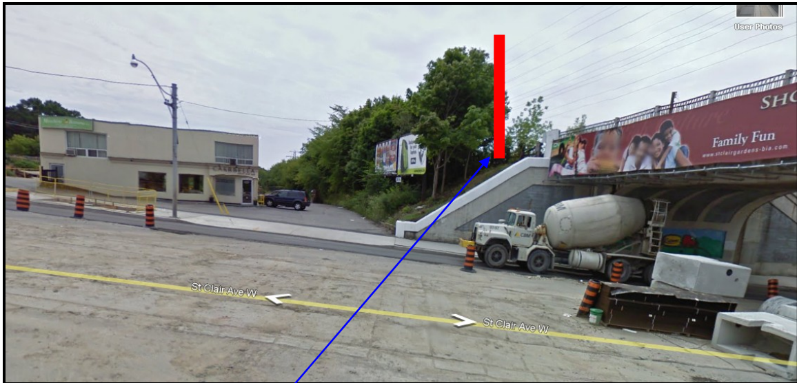
South side of St Clair Ave W, looking at the existing billboard signs on the east side of the rail line, which is to be removed.
