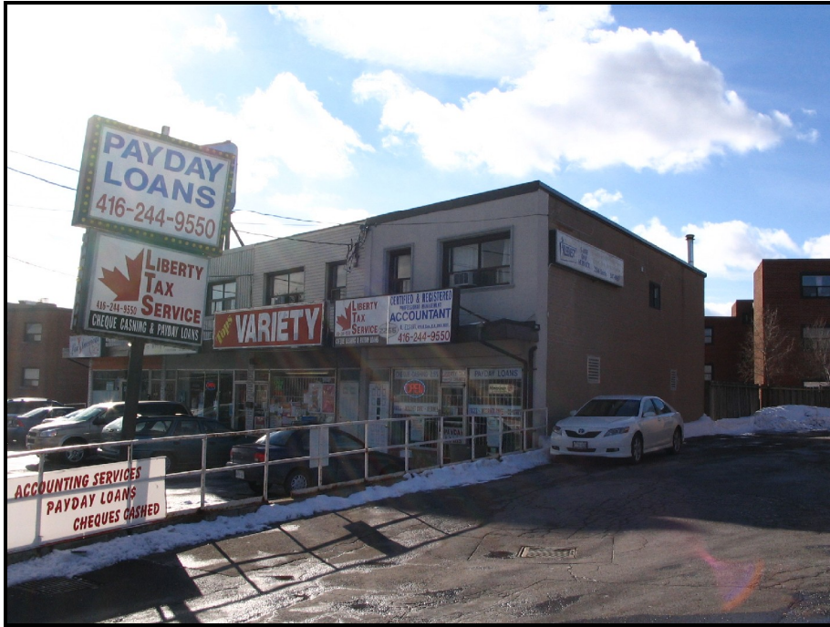
2266 Keele St - North end of a strip of 4 buildings. Picture taken before the erection of the tri-vision roof sign.
