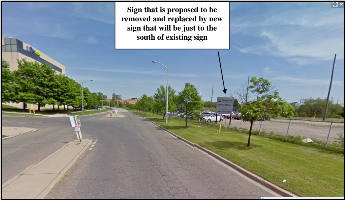
Continuing to look north along Galaxy Blvd from the foot of International Blvd.
