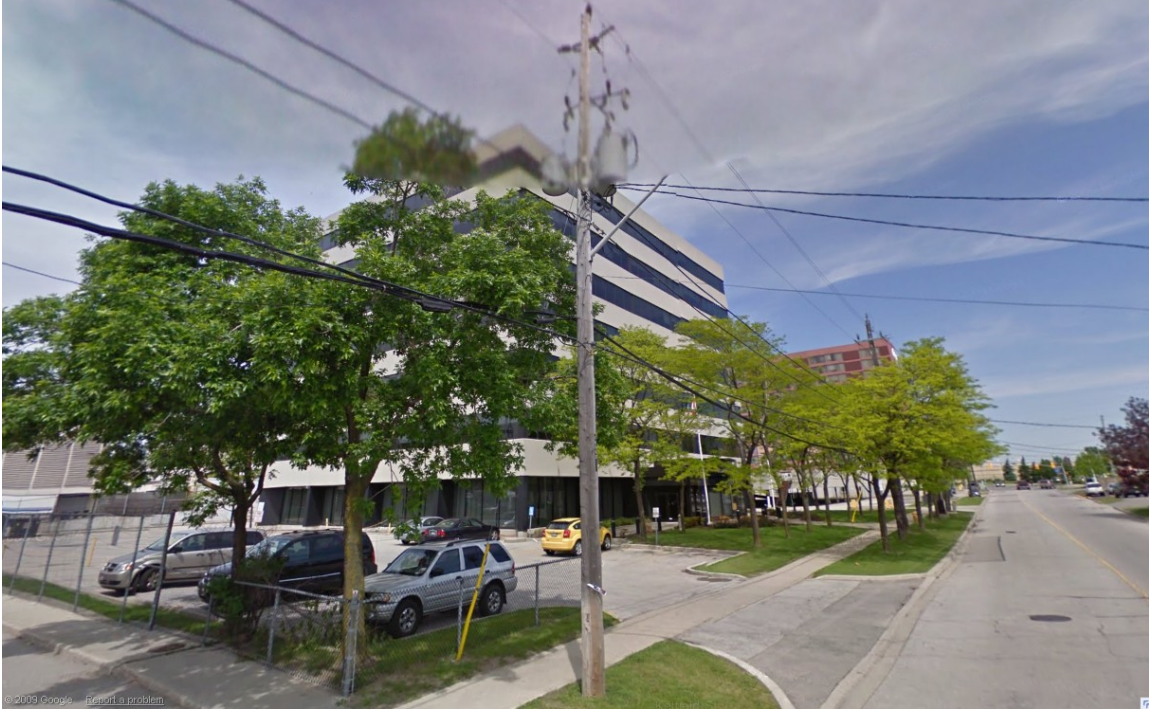
Entrance off Kelfield Rd onto the property of 655 Dixon Rd looking north towards Dixon Rd
