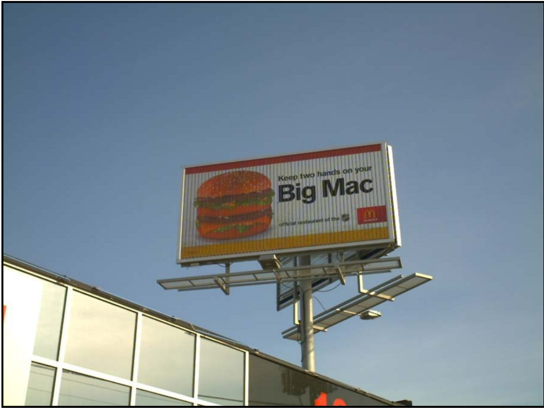
Existing Sign – East Direction
