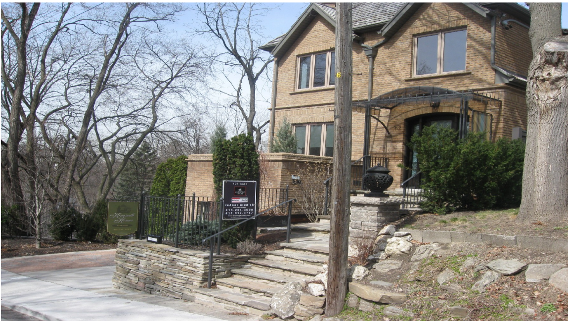
Photo 2 – Showing new stone retaining wall and wrought iron fence/guard
