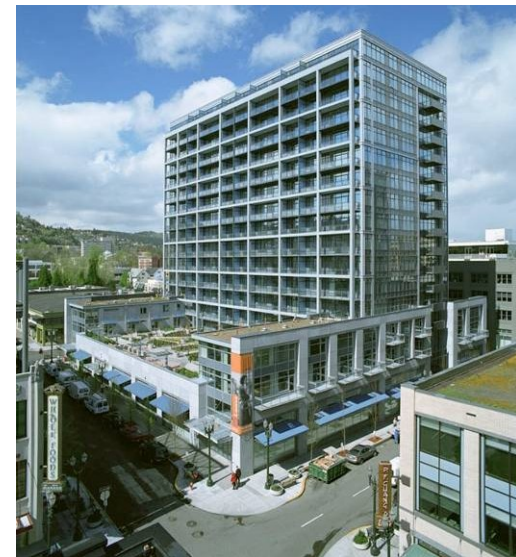
Figure 32 – Base building massing to create a pedestrian scale street space
