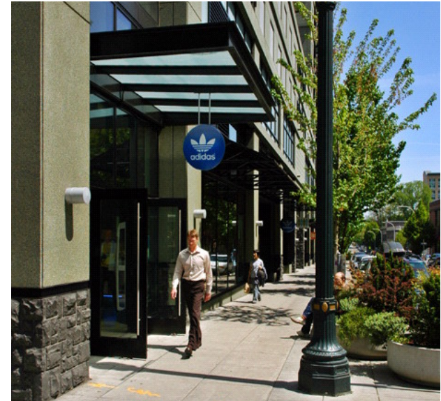
Figure 30 - Canopies and glazing at street
