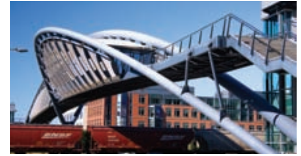
Amgen Helix Bridge - Seattle, Washington
