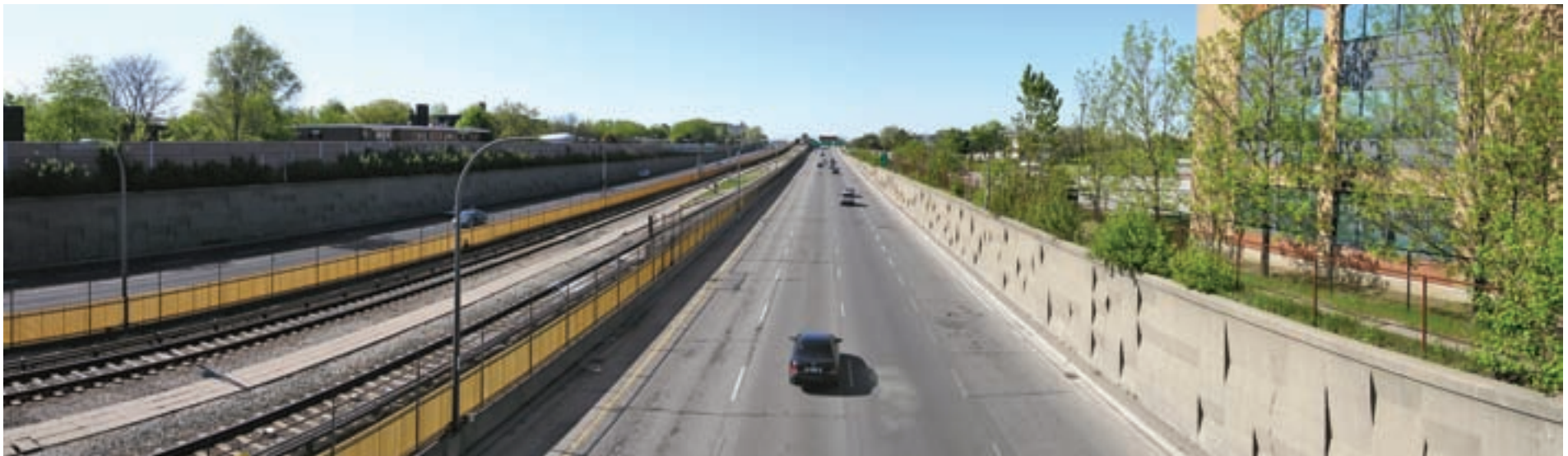
Allen Road looking north from Flemington Road bridge
