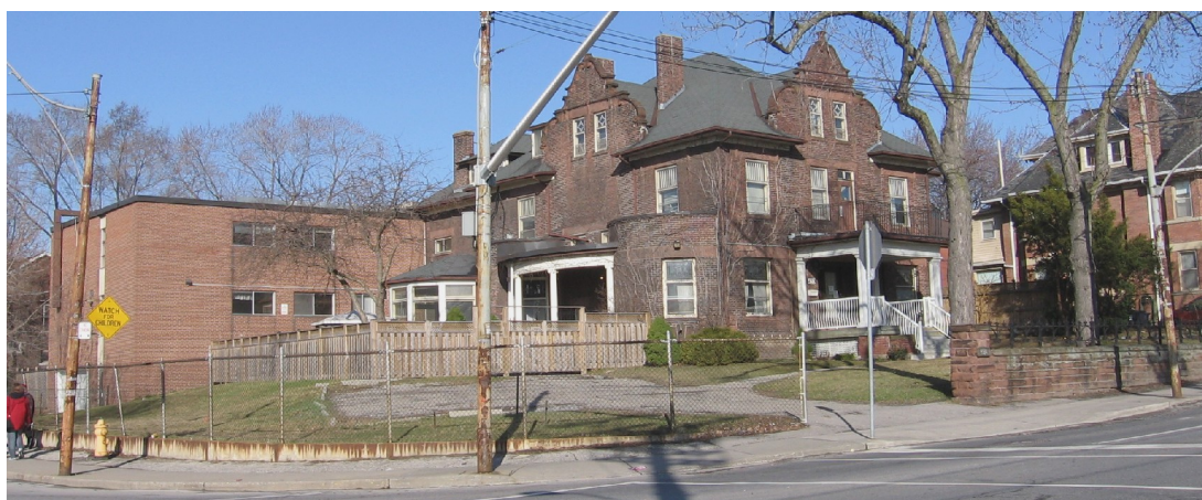
View of the principal (east) façade facing Pape Avenue (right) and the south elevation overlooking Riverdale Avenue (left)
