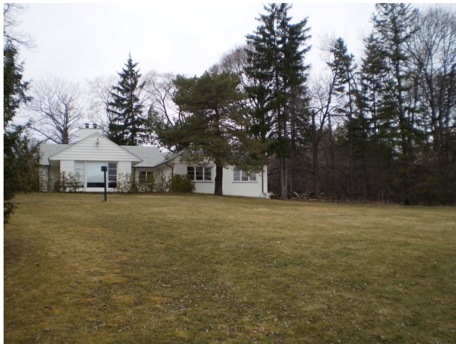
2489 Bayview Avenue showing the rear of the gatehouse (east façade)
