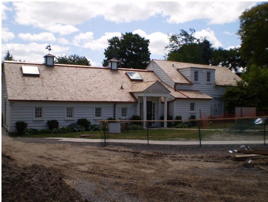
2489 Bayview Avenue showing the stables (north façade)
