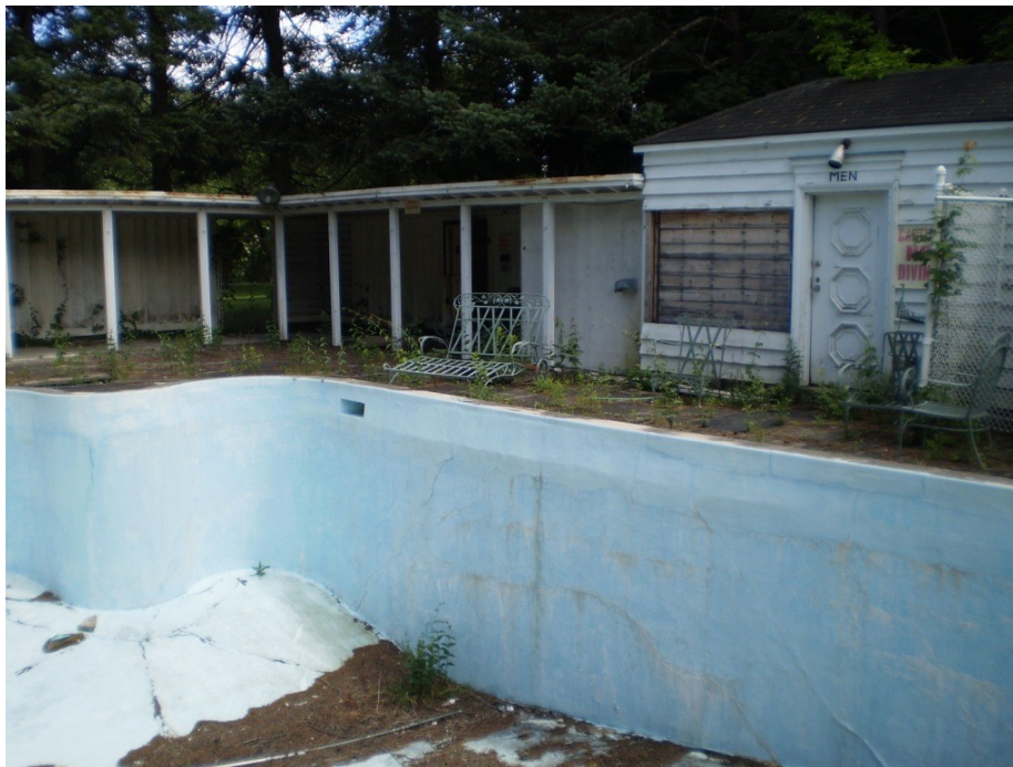
2489 Bayview Avenue showing the pool, and cabana deterioration
