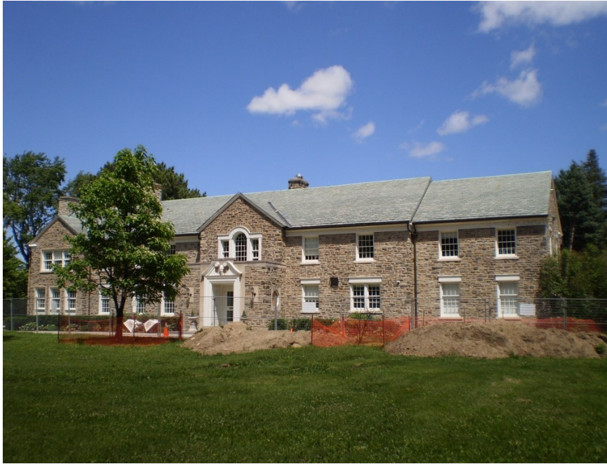
2489 Bayview Avenue showing the main house (west façade)
