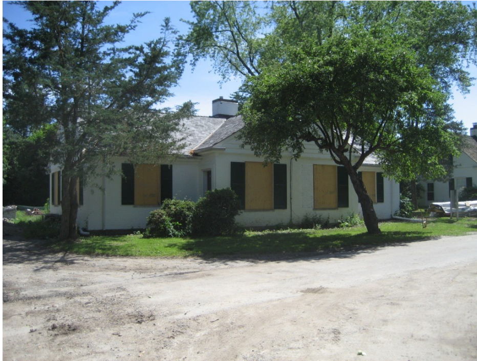
2489 Bayview Avenue showing cottage a/b (east façade)
