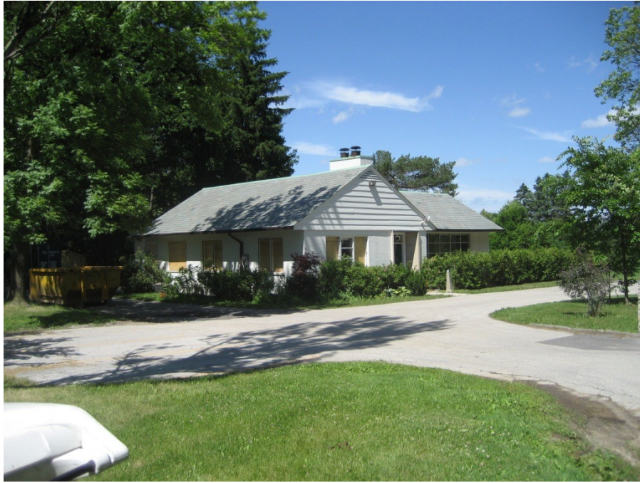
2489 Bayview Avenue showing the gatehouse (southwest façade)
