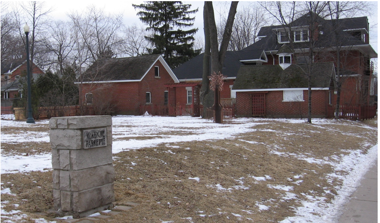
McKenzie Parkette, looking south and showing the Stable (left) and Milk House (right), with the John McKenzie House and Carriage House in the background
