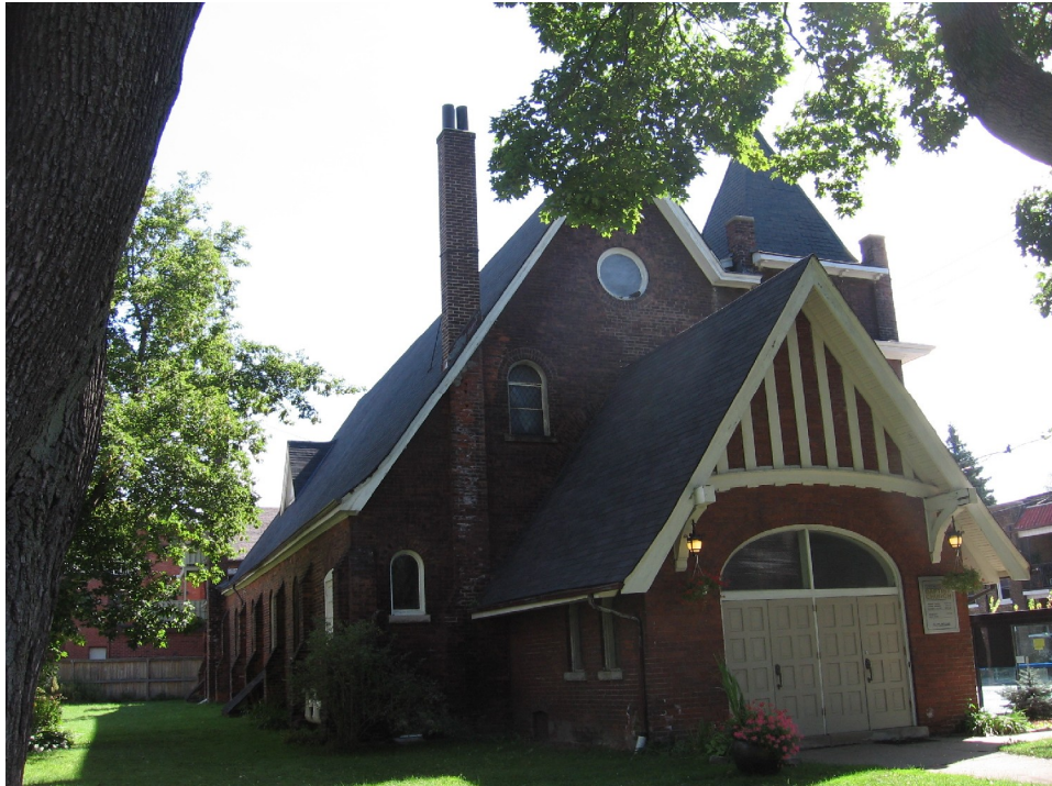
North and west (main) elevations
