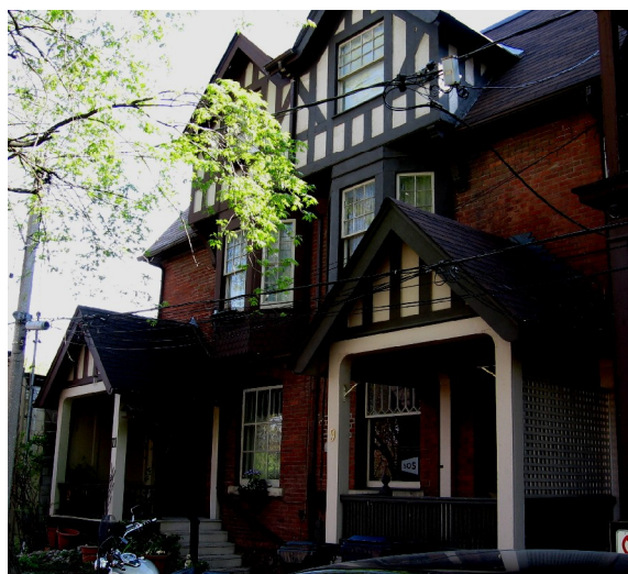
Right: 9-11 Edgedale Road
