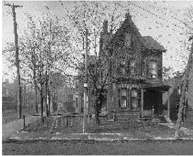
View of the west side of Glen Road at Howard Street in 1913, with the properties at 2 Glen Road & 8 Howard Street (left), and showing the east façade of the William Muir House at 2 Glen Road (Source: City of Toronto Archives, Fonds 200, Item 70, March 14, 1913)
