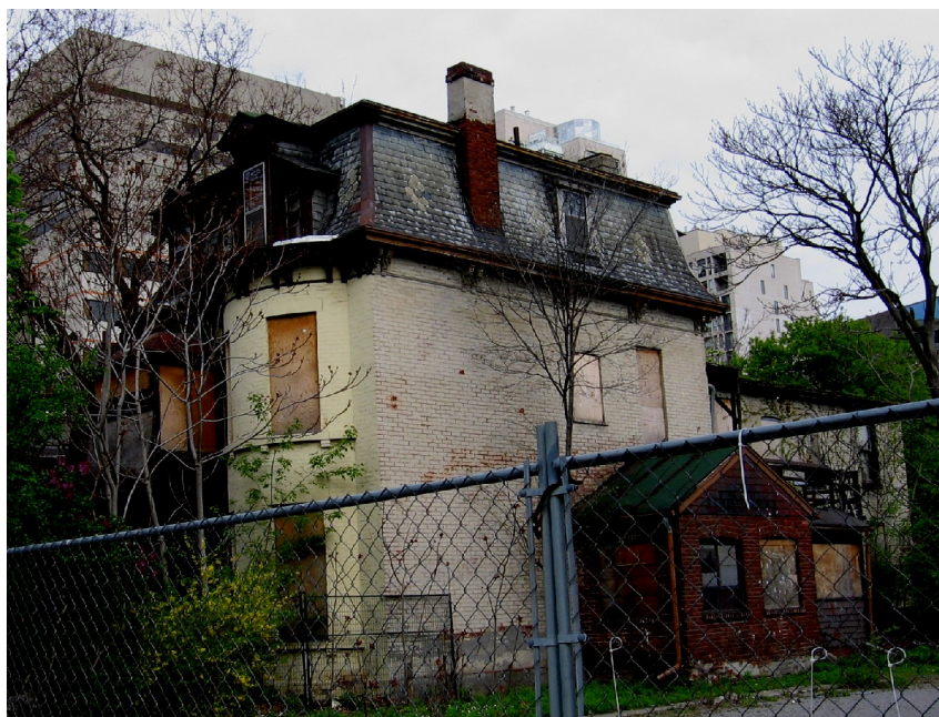
Photograph showing the south (left) and east (right) elevations of 4 Howard Street, 2010
