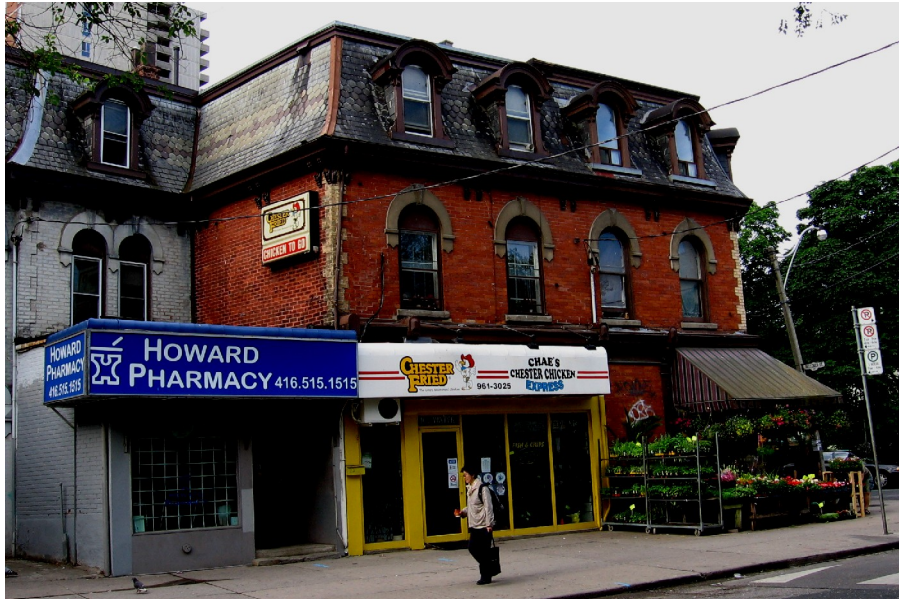
Photograph: 21-23 Howard Street (right), with 25 Howard Street on the left (April 2010)
