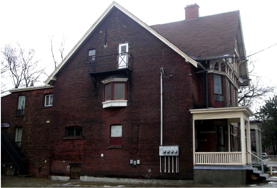
Photograph of the west elevation of 32 Howard Street, April 2010
