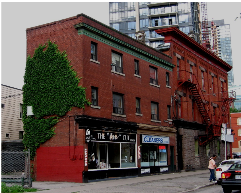
View of the north elevation on Howard Street with the rear (east) wing
