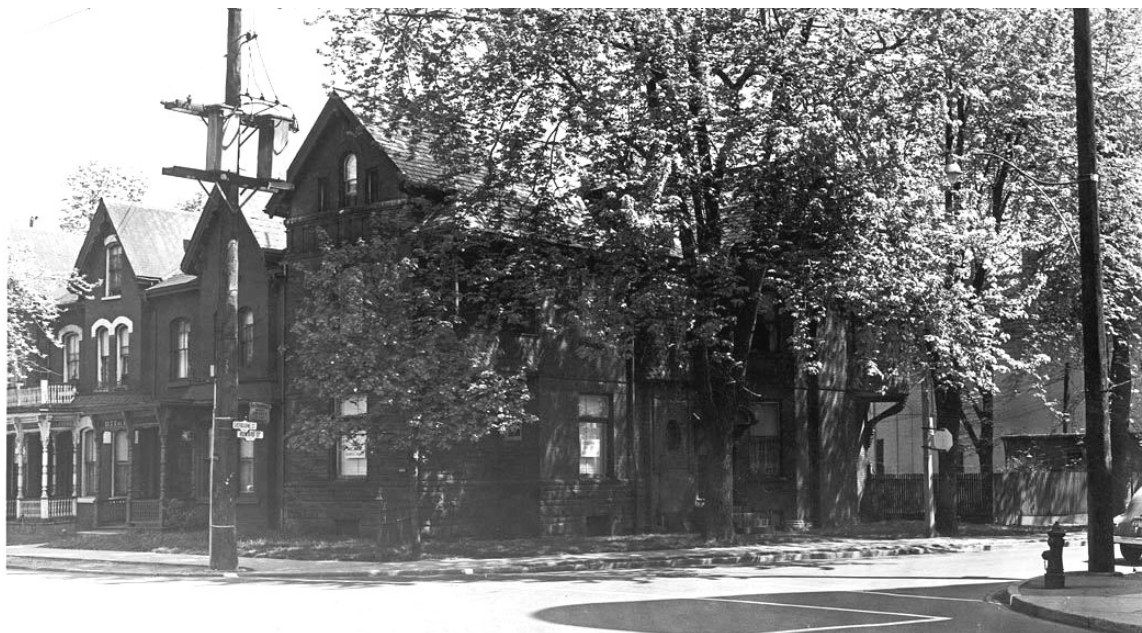
Anson Jones House at 603 Sherbourne Street in 1953 (Source: City of Toronto Archives, Fonds 200, Item 387, May 12, 1953)
