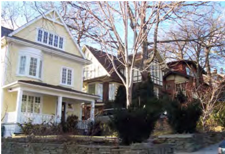
Figure 3. South Kingswood Road, west side, #38, #40, #42
