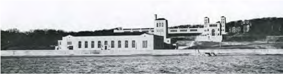
Figure 11. Victoria Park Pumping Station, December 17, 1936.
