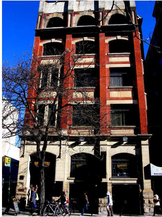
Principal (south) façade of the Nicholls Building
