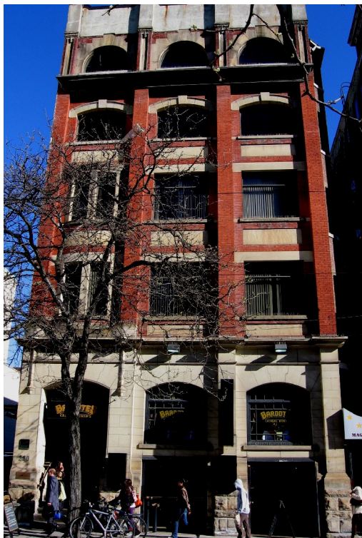
South facade of the Nicholls Building
