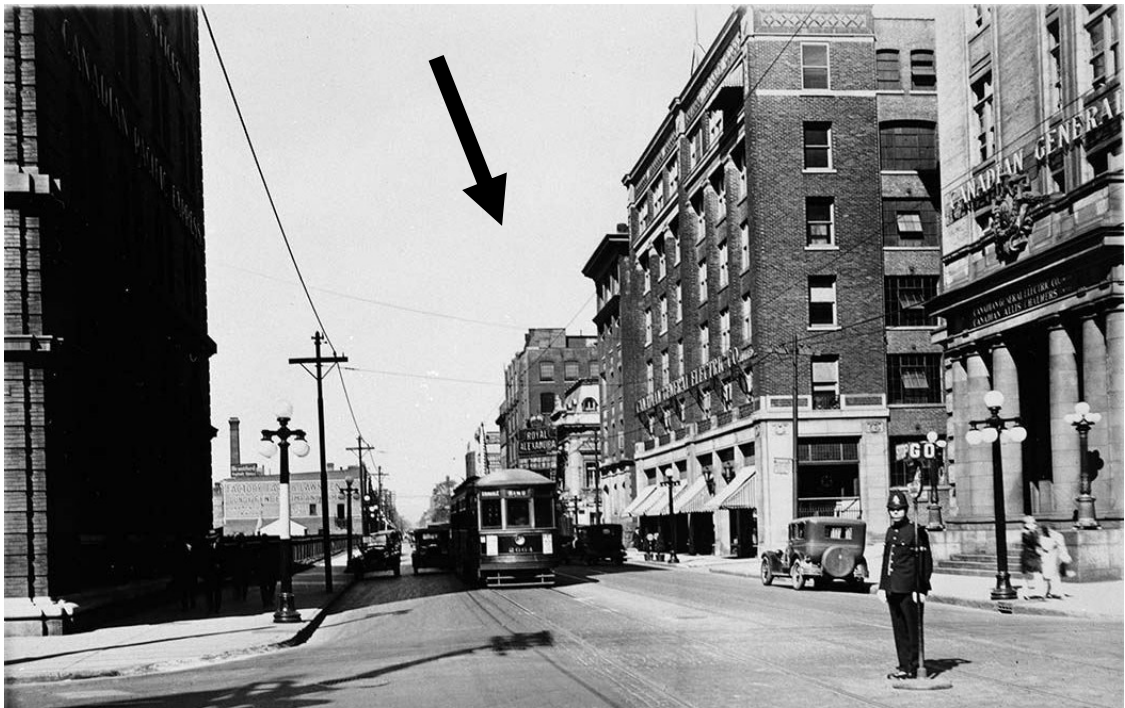
View of King Street West, looking west from Simcoe Street, and showing the Nicholls Building mid-block in July 1927 (Source: City of Toronto Archives, Fonds 1231, Item 2165)
