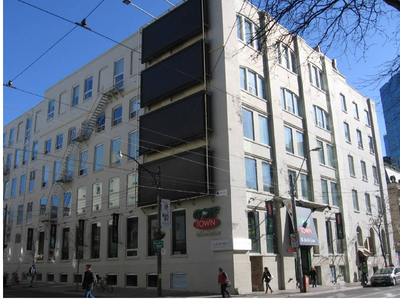
Photograph of the Reid Building at the northeast corner of King Street West and Ed Mirvish Way, showing the south (right) façades of the 1904 (centre) and 1913 (right) warehouses, with the north warehouse (1909) visible on the far left
