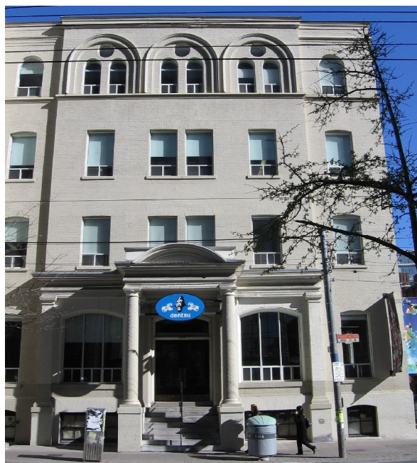
Principal (south) facade on King Street West of the Gillett Building (1901)
