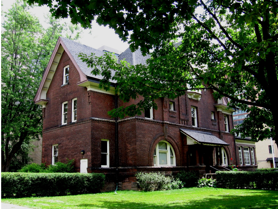
1 Elmsley Place, showing the principal (west) façade (right), July 2010
