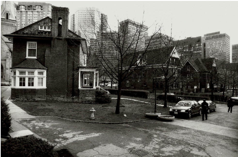
5 Elmsley Place (left), with #3 (centre) and #1 (right) from the Heritage Easement Agreement, 2000
