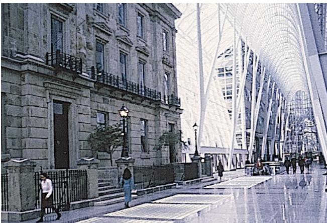
"The Galleria", Santiago Calatrava
