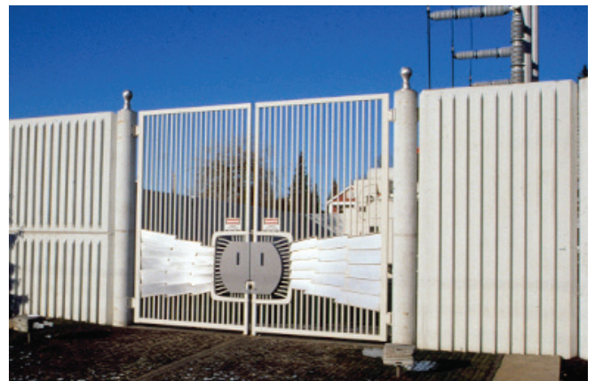
“Gate, electrical substation”, Clair Colquitt – Seattle
