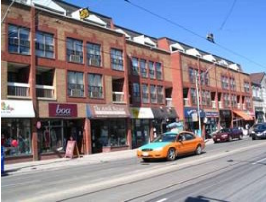
The mass of this building is broken up vertically by providing distinct building base, middle, and top. It is also divided horizontally along the street frontage with recesses and regular vertical articulations.
