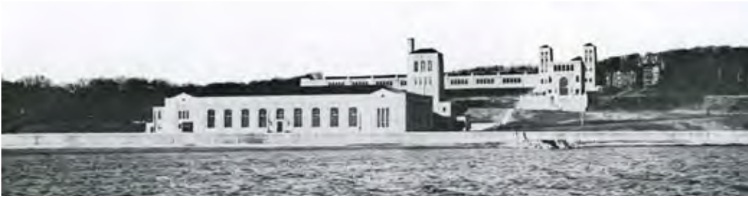
Figure 11. Victoria Park Pumping Station, December 17, 1936.
