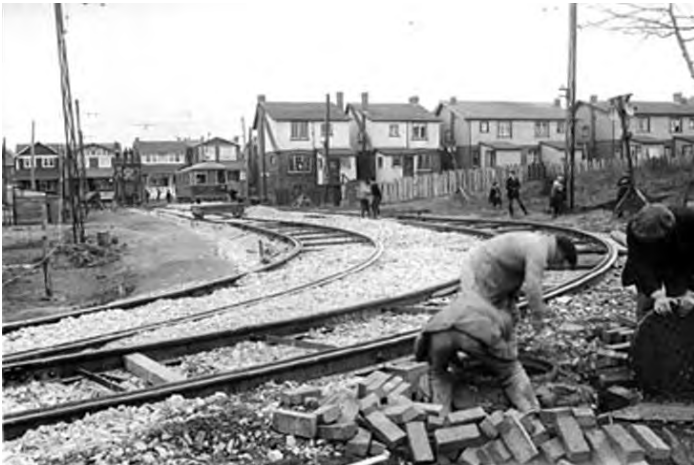
Figure 10. Construction of the Bingham Loop in 1922
