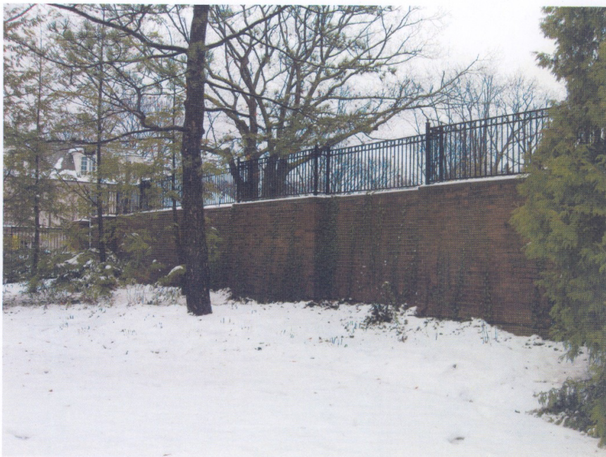
Attachment 3, Photograph of wrought iron and brick wall fence, South side
